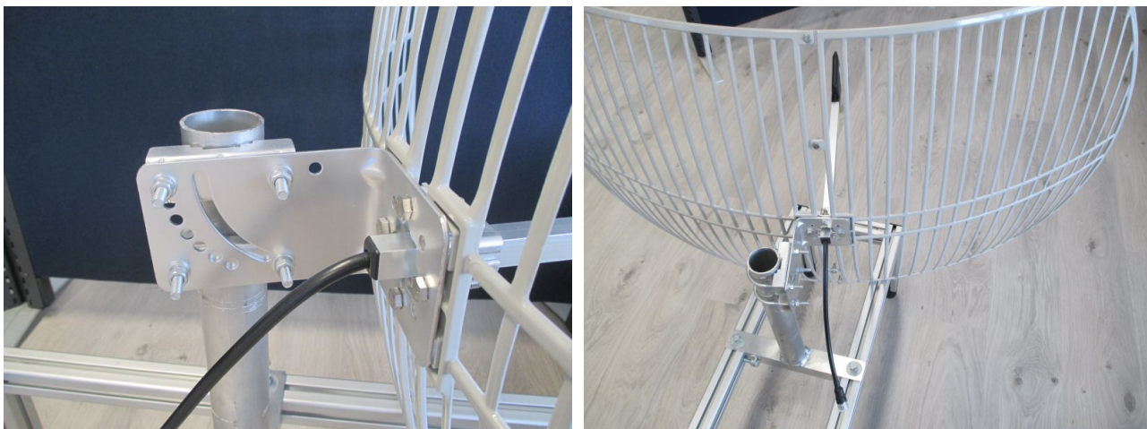
Figure 13: Step 4 – Fix the antenna to the supporting pole
