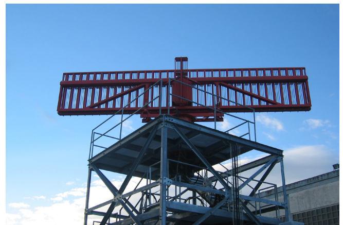
Figure 4 | Standalone En-route SSR antenna installation (without co-located PSR) Source: Intersoft Electronics NV
